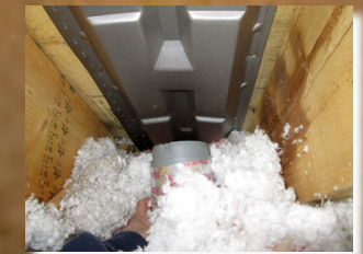
Bathroom exhaust discharge buried but not connected to exterior of home.
