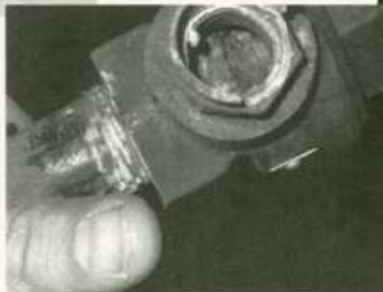
(Above) Lifting the handle of a pressure relief valve to check for proper operation
